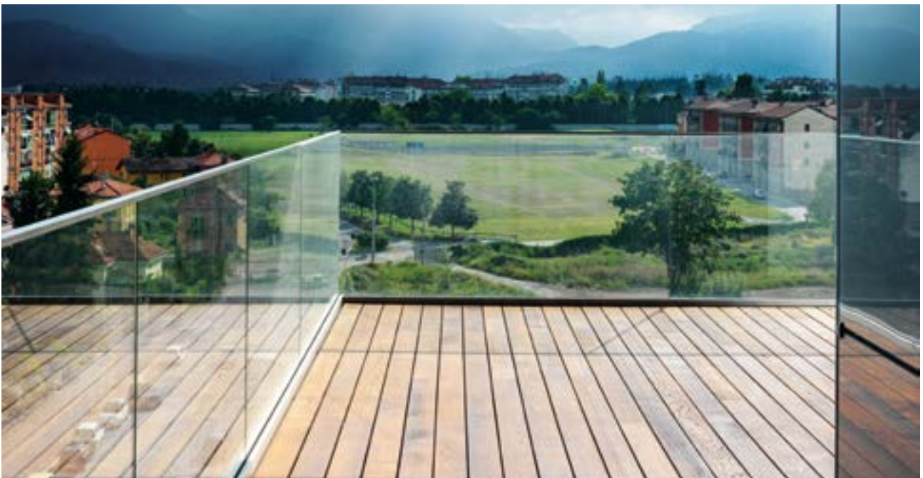
F5 Multifunctional building, Cuneo
