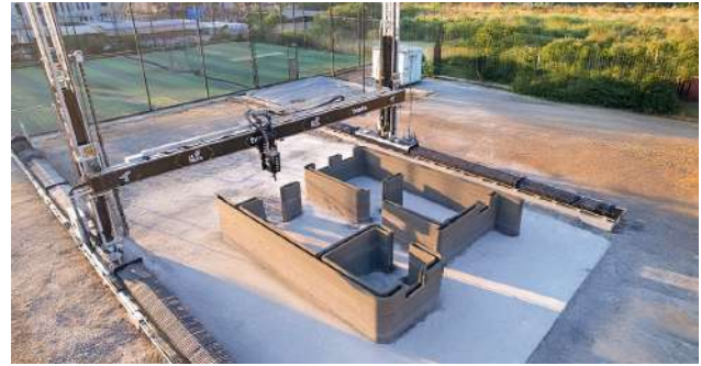
Photos above and right: The Cedar 3D Concrete Printer. Photo credit: Tvasta
