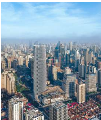
Best Tall Building, by Region, Asia Pacific Xintiandi Commercial Center, Shanghai, China (Photo credit: Shui On Land)
