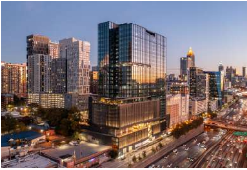
Best Tall Building, by Region, Americas 1020 Spring Street, Atlanta, United States (Photo credit: Gregory Campbell, Portman Holdings)
