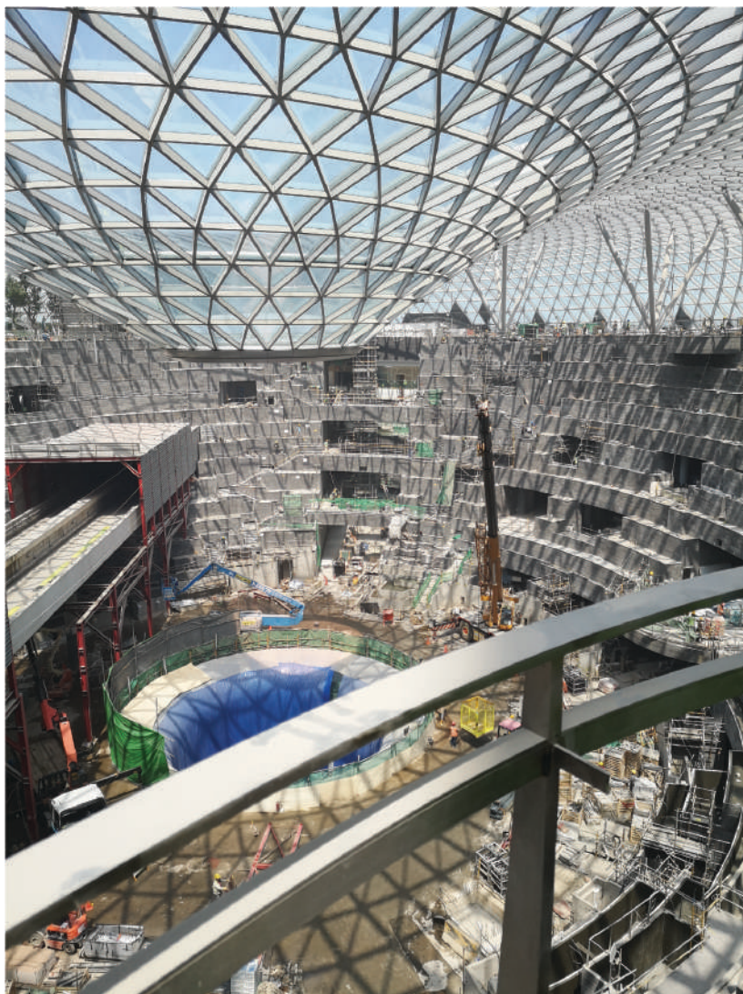
Photo 2: Shiseido Forest Valley (Construction Phase). Photo: Sika
