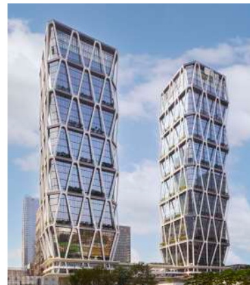
Best Tall Building, by Region, Asia Sany IROOTECH Headquarters, Guangzhou, China (Photo credit: Dave Burk, SOM)
