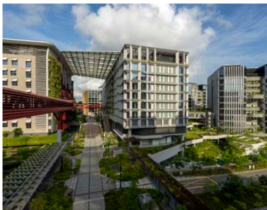
Best Tall Building, by Region, Asia Punggol Digital District, Singapore (Photo credit: Darren Soh)
